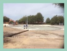
We are currently 4 weeks into the car park extension works programme with most areas now excavated and filled with new aggregate to the designed build up. The ACO drainage and pin kerbs are currently being installed, along with the oil separation tank for preventing polluted waste entering the main drainage run to the road. We will shortly have the electric cabling installed for the lamp-posts so we are prepared for the tarmac.
