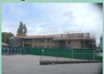
The external Brickwork to the East elevation is the first side of the building to be successfully completed allowing the scaffolding to be stripped, it's exciting to be able to finally see the appearance of the building. We will have all elevations completed by the end of July so we can strip the remaining scaffold and focus on installing the windows and doors. The photo above presents a visual of the west elevation brickwork nearing completion.
